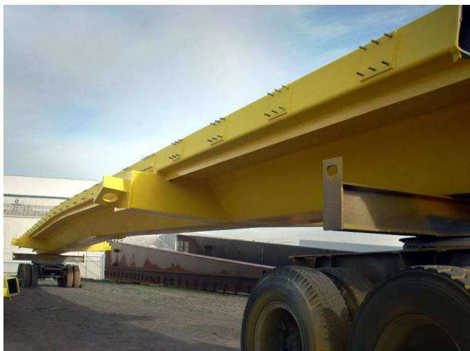
Clarks Lane Cable-stayed pedestrian bridge ready for transportation
