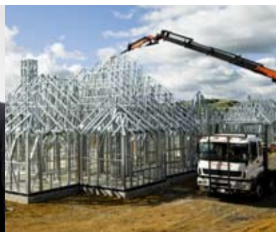
Steel framing being erected in Ramarama in South Auckland
