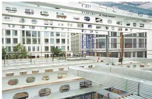
An example of Fabsec beams with intumescent coating applied off-site
