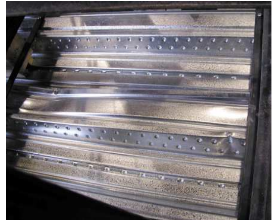
Deformation in the mid-span region of the floor deck test specimen at maximum load
