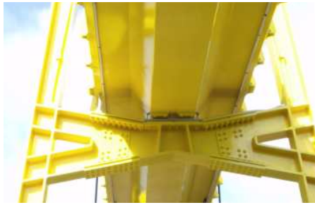
Clarks Lane footbridge, a cable stayed steel box beam with in situ concrete deck, over new SH18 Hobsonville Deviation which opened August 2011. Designed and built by HERA members Jasmox, Jeff Wells, Aurecon, Eastbridge and HEB Construction.
