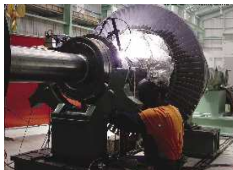
Repair of extensive erosion damage to turbine rotor labyrinth diameters, built up with Inconel 625, by HERA member Allied Industrial
