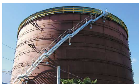
Tank fabricated by HERA member Page & Macrae with stairs manufactured by HERA member Mobridge
