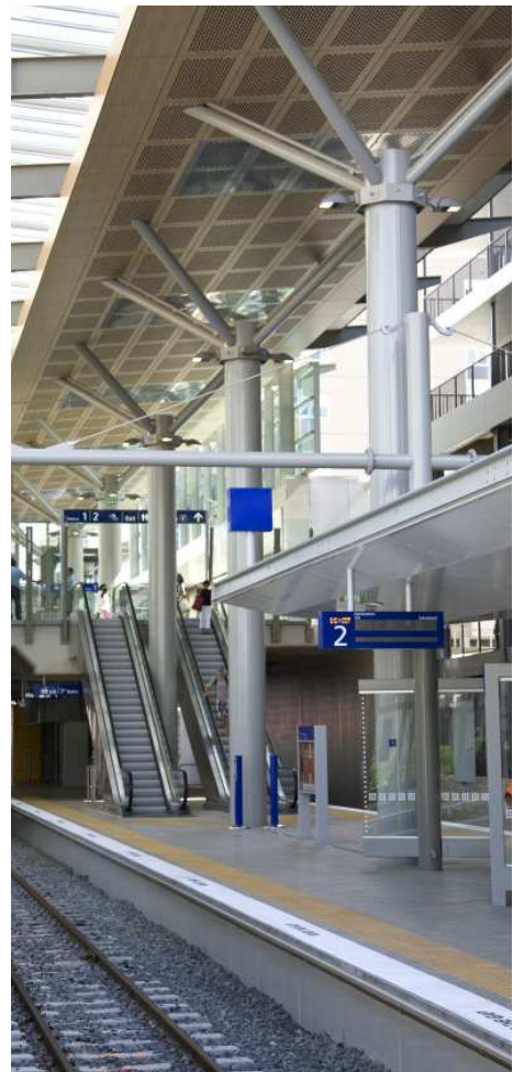
Auckland New Market southern concourse railway station undertaken by HERA member GGE for Hawkins Construction with glass-finished paint systems, interconnecting links. The roof sections shown were erected during night hours, assembled on-site upside down, then flipped upright and hoisted upon the columns.
