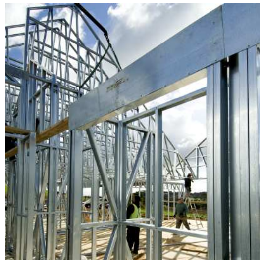
HERA is contributing to light steel framed housing technology development, a construction system which steadily increases its market share
