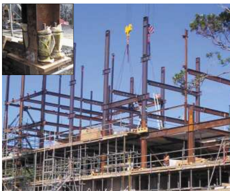
HERA seismic design solutions are now in every multi-storey building in New Zealand. Aurecon's International Structural Engineers UK award-winning Te Puni student accommodation building is shown here. It incorporates damage avoidance systems such as rocking frames (shown inset) and sliding hinges
