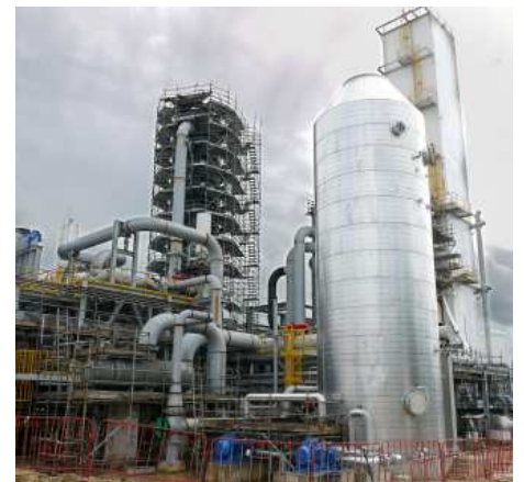
Oxygen processing plant built by HERA member Tenix New Zealand for the Lihir gold mine on Lihir Island, PNG
