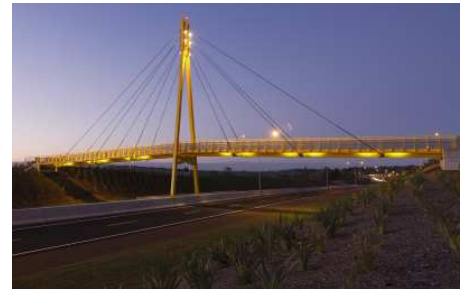
Clarks Lane footbridge, a cable stayed steel box beam with in situ concrete deck, over new SH18 Hobsonville Deviation which opened August 2011. Designed and built by HERA members Jasmox, Jeff Wells, Aurecon, Eastbridge and HEB Construction.
