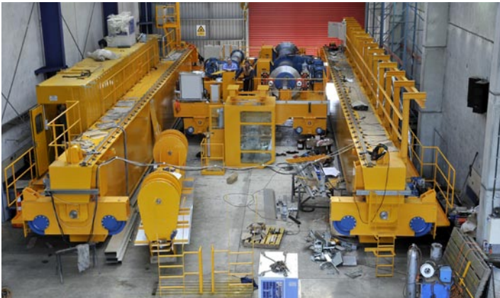
HERA member JJ Niven Engineering manufactured the major structural components and conducted assembly of a 100/30/5 tonne x 19.8m span overhead travelling hot metal crane for Pacific Steel's plant in Auckland. The crane would be the largest hot metal production crane in New Zealand. Even more impressive is that it is made with local capability and expertise, despite competition from cheaper imports.
