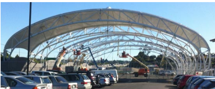
HERA member Structurflex was the designer and build contractor for this elegant solution for a school sports venue, while HERA member Graysons Engineering was fabricator. The design is a great example of how lightweight PVC membrane /ETFE foil, supported over an elegant steel structure with galvanized steel cables, could provide substantial cover (2450m 2 plan area).
