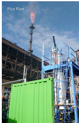
Left: Green steel innovation LanzaTech Pilot Plant at NZ Steel – NZ Steel and biofuel company LanzaTech struck a deal to extend their 2008 pilot project to convert waste gases into low carbon fuels
