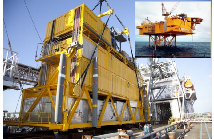
HERA member Fitzroy Engineering's export success: The 650 tonne, $36 M Yolla module on its way to the Bass Strait – Fitzroy also won the actual installation job. Inset: Yolla MLE Accommodation & utilities module in place on the Yolla gas platform, Bass Strait, Australia
