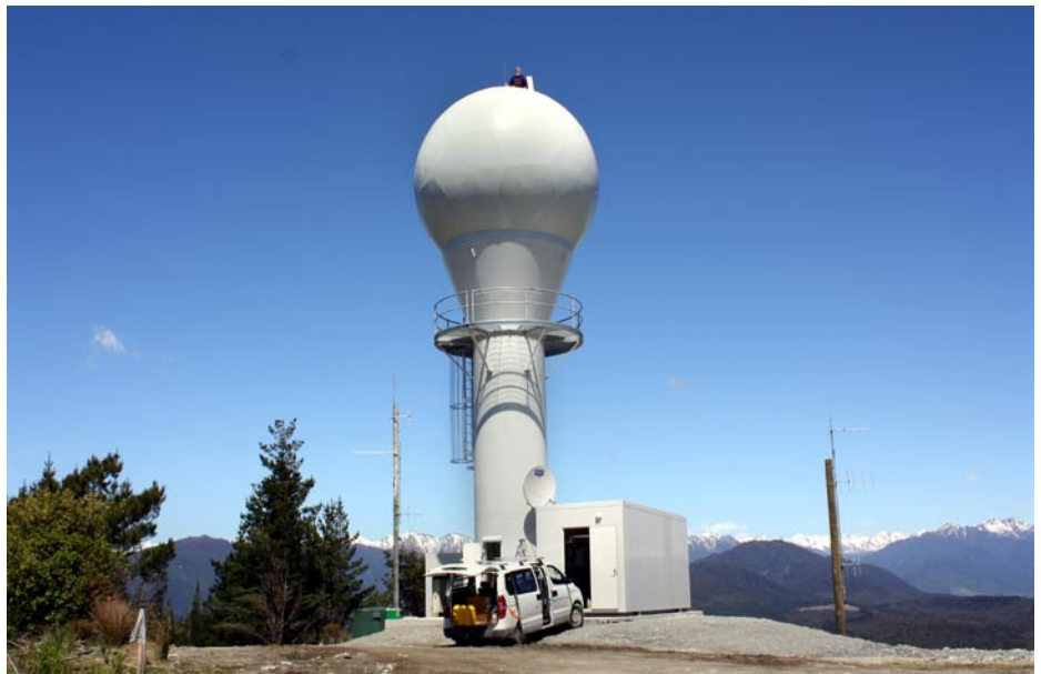
HERA member Acme Engineering fabricated and erected this rain radar tower for the NZ Meteorological Service just outside of Hokitika
