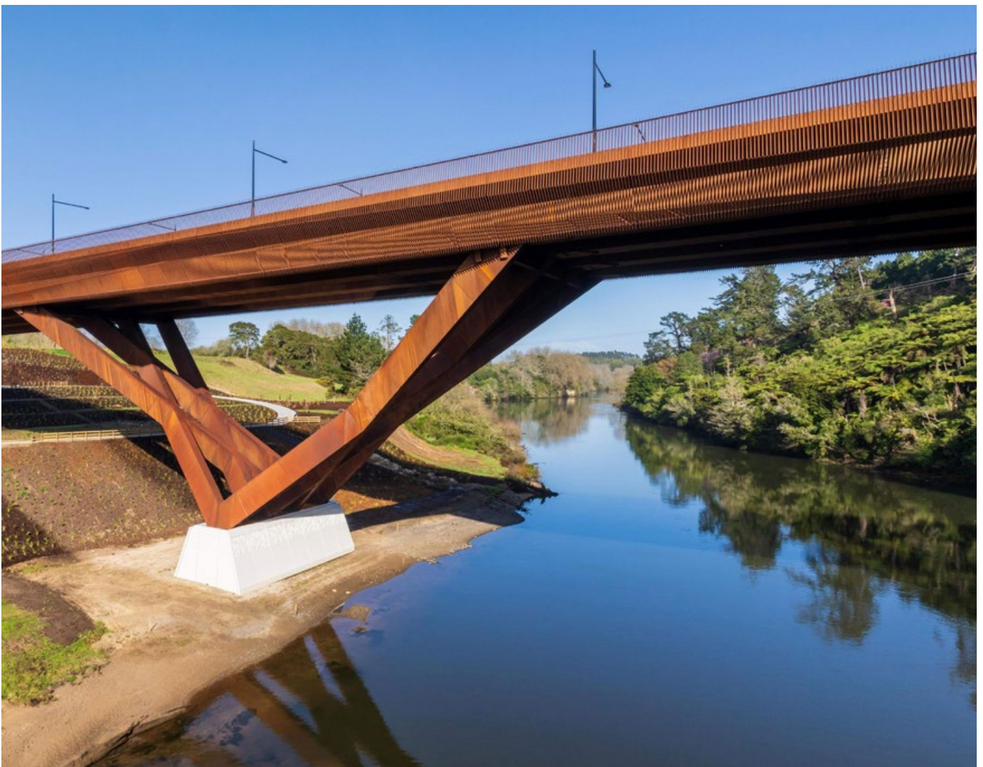
Courtesy of BBO, Side view of Te Ara Pekapeka Bridge substructure looking towards the Southern abutment
