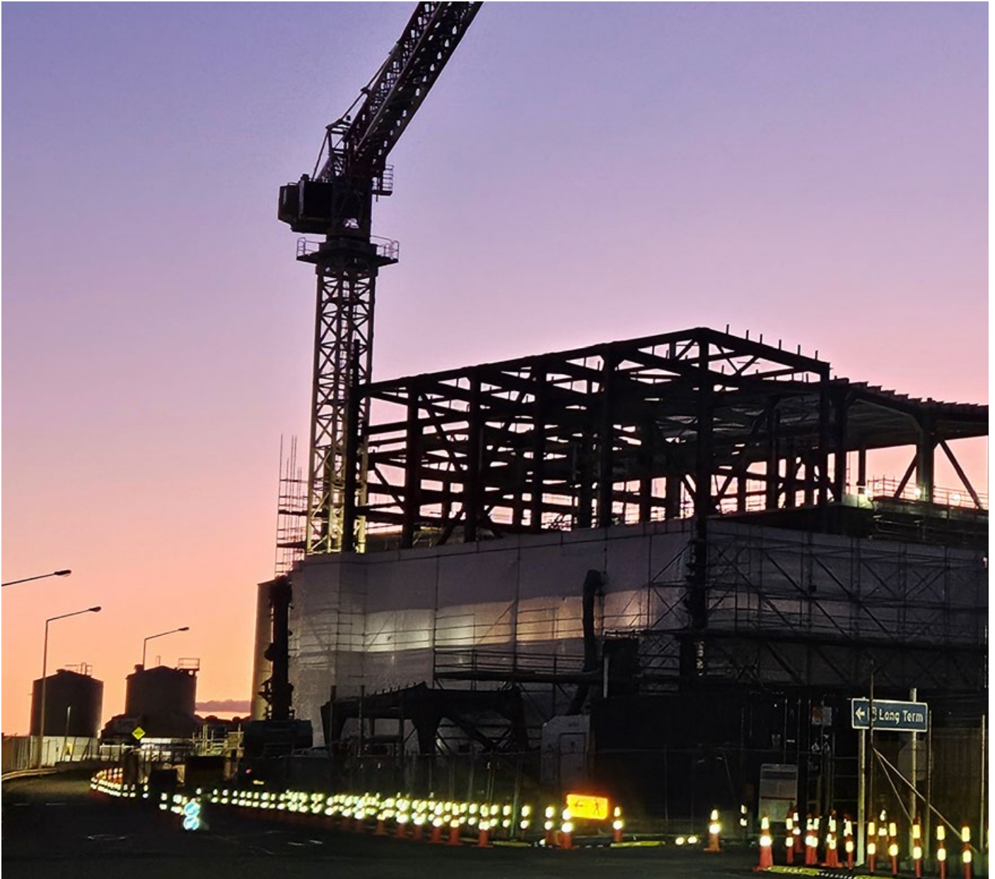
Courtesy of MJH Engineering Ltd., Te Whare Wai Para Nuku, Wellington
